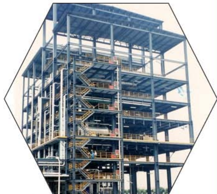
Nantong Jiangtian Chemical Co, China 10000 TPA capacity
